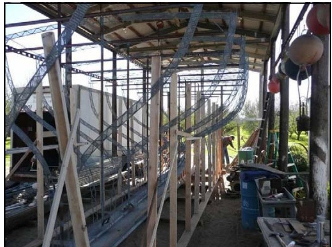
Installed: The vertical frames.
