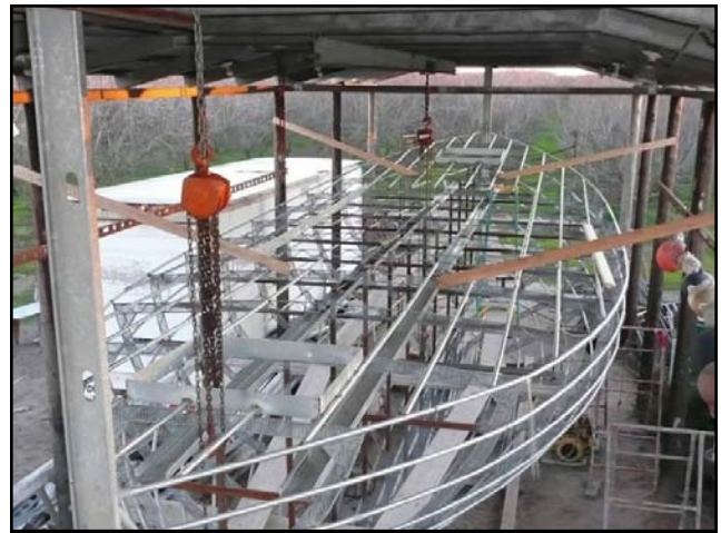
Deck Pipe and Hatches: Now installed.
