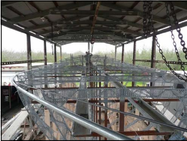
Deck Frames: Now in place.
