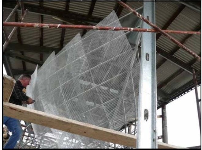
First layer of lath.
