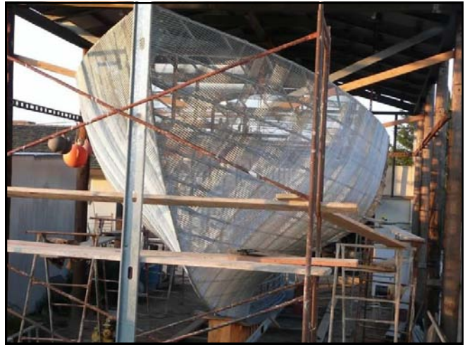
Bow View: Finished layer of lath.
