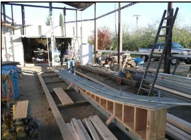
The beginning: Setting the centerline
